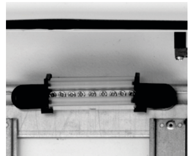
Patented IP2X neutral terminals with flexibility to position it on the chassis
